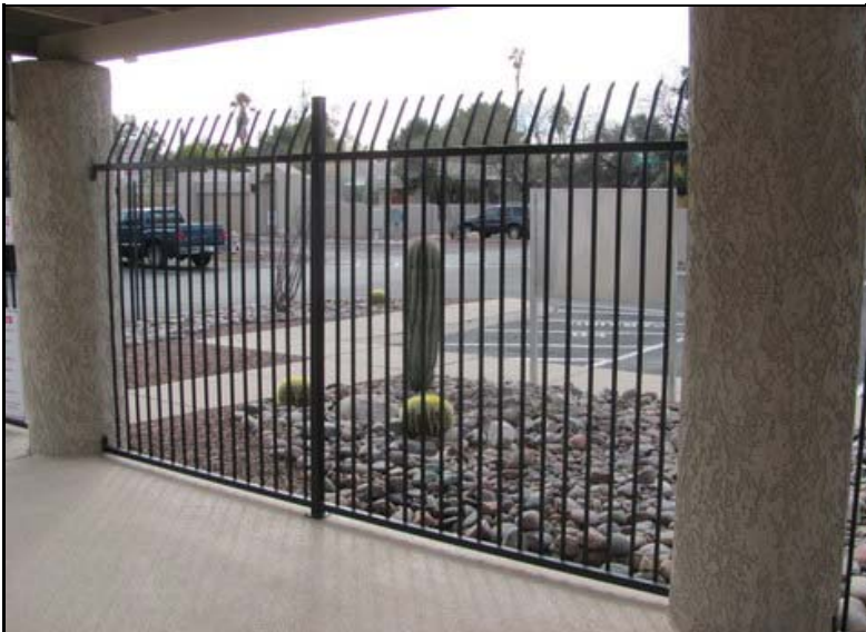
Metal pool fence
