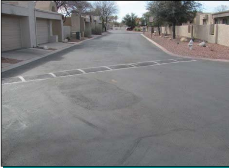
Asphalt pavement overview
