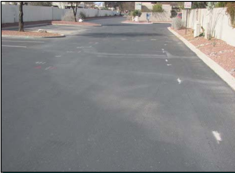
Asphalt pavement overview, Bullrush Lane
