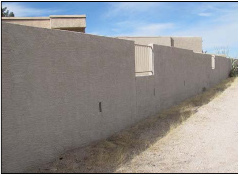
Perimeter wall overview
