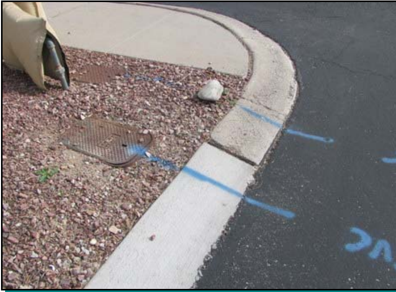
Previously replaced and original concrete gutters
